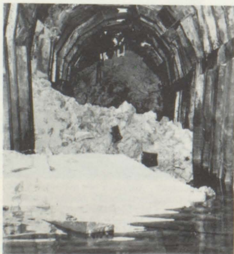
Top, Mike Neises inspects one of several serious cave-ins in the tunnel. Right center, many of the 12x12 redwood timbers are beginning to give way after 95 years. Page center, Alpine Tunnel station is being restored by the Gunnison Historical Marker Project. Upper left, Aspen were beginning to turn hints of gold at the time of the September trip. Left the tunnel is blocked for about 200 feet near the east portal and water is backed up about 2 feet deep. Above, about a mile of the railroad grade can be seen where it crosses the sheer face of the Palisades on 550 feet of stonework buttressing. The tunnel is considered an engineering marvel even today.
