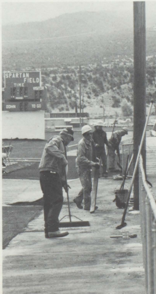
THERMO PANE WINDOWS were installed in Kesner Jr. High to help cut heating costs (above). Addition of asphalt in front of the grandstands on Spartan Field was part of the solution to drainage problems. New sod, removal of the old track, and crowning of the field were also included in the project.
