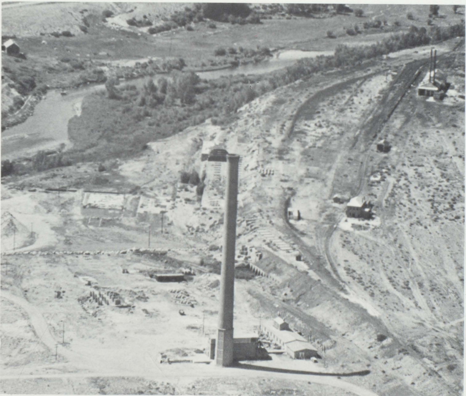
This aerial view of the smokestack shows the site that was considered in 1902 to be an "ideal spot two miles from the business center of Salida."
