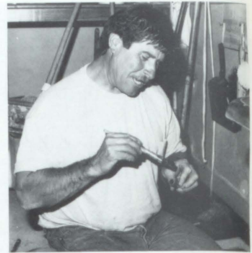
FEW PEOPLE were thirsty Oct. 15, until it was announced that all water was shut off. A pipe burst in a Kesner Junior High closet and when the door was opened, there was a flood. Maintenance man Gene Guccione said they had to do the quickest thing possible - shut off the water.
