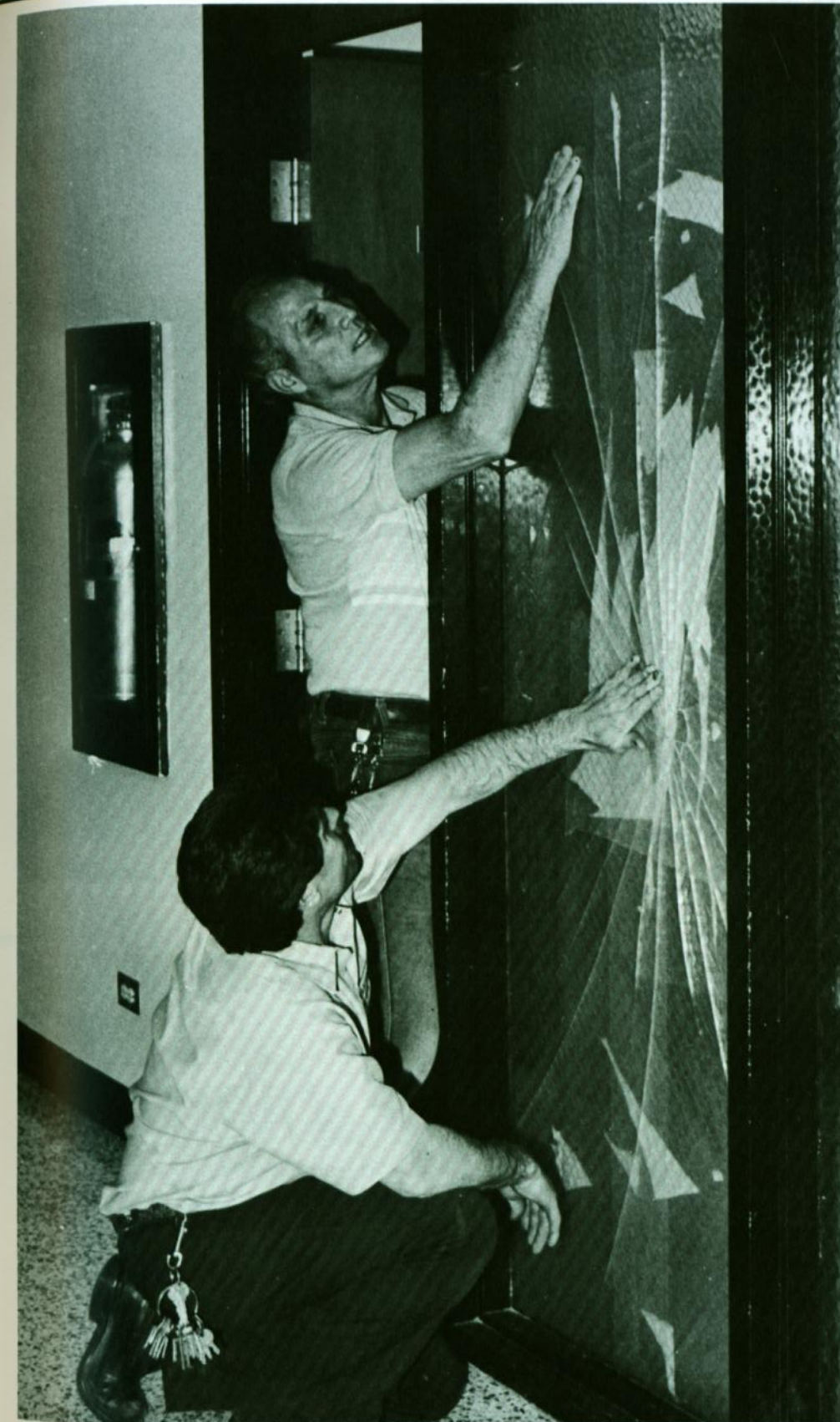
TEMPORARY REPAIRS were necessary March 30, 1988 when the window in the work room in the academic hall was broken by two scuffling high school students. Charlie Cribari and Gene Guccione put large tape on the glass to keep it from falling out. Cribari estimated damage at about $300 for parts and labor.
