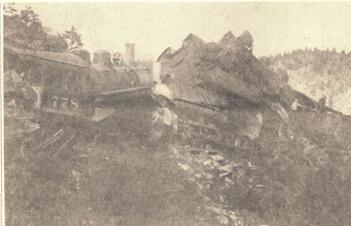
HEADON CRASH — Thirty years ago trains No. 7 and 8 collided a mile and a half east of Granite. No. 7 was a double header, and both were passenger trains. Firemen on each train were killed. The tragedy was blamed onto human error. A detailed account of the wreck appears on this page.
