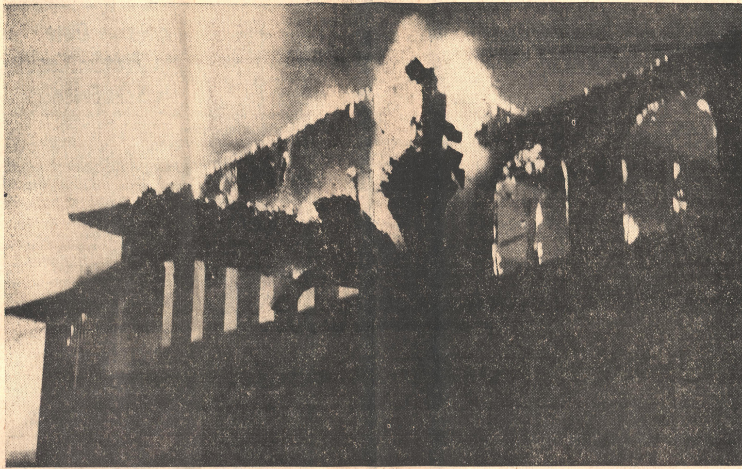
EAVES COME CRASHING DOWN—Before dawn Saturday, a fire which reportedly started at 3:30 a.m. in the office of the main Salida high school building had raged upward, destroying the roof entirely and sending the eaves crashing down to the sidewalk below. Mountain Mail Photo
