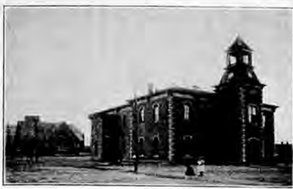
D Street Public School and Methodist Church.
