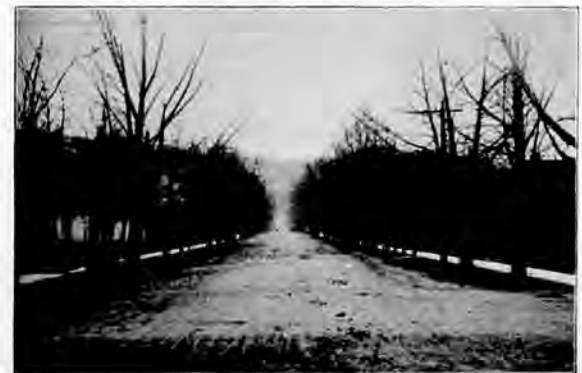
Looking Up E Street.
