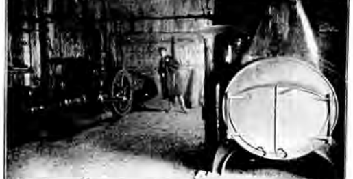
Interior of Machinery Room.
