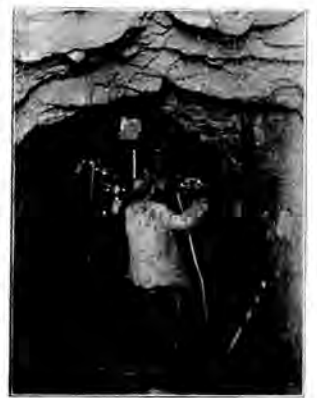
Breast of the Tunnel.
