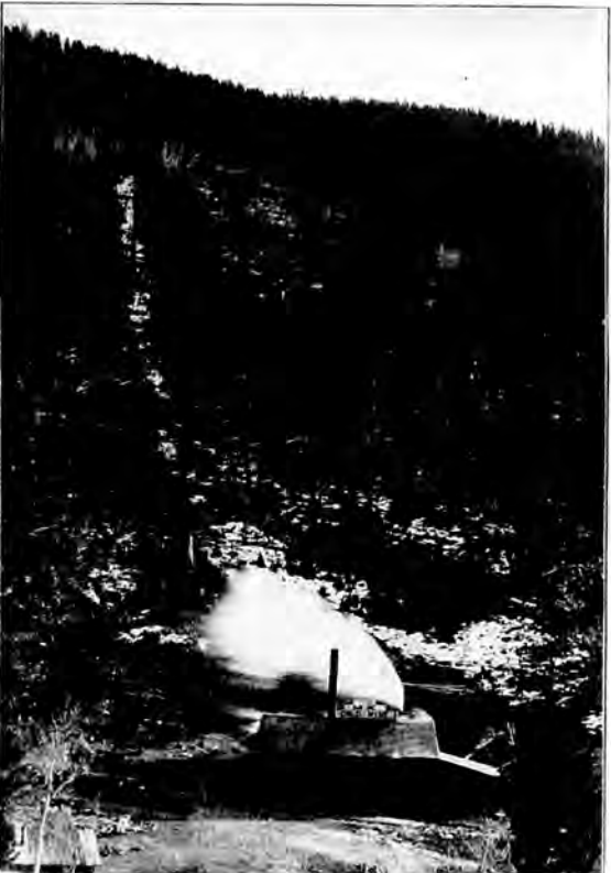
Great Hershberger Tunnel Site and Cameron Mountain.
