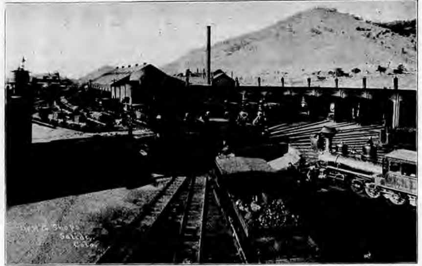
View of the Rio Grande Yards, Showing Narrow Gauge Round House and Shops.
