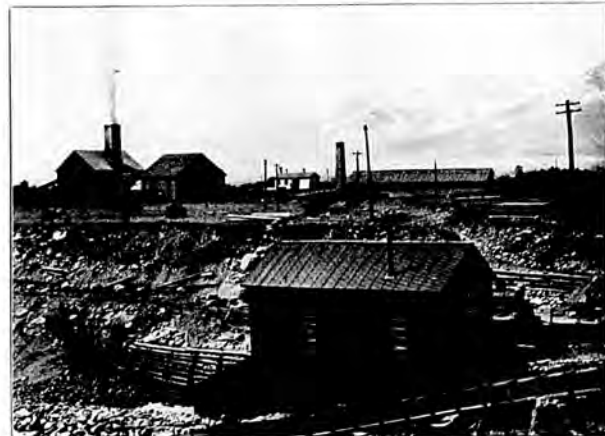
The Buena Vista Smelting Works.
