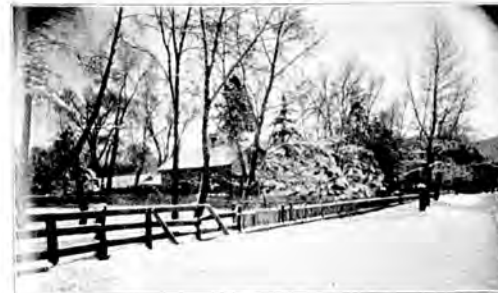
Residence of Hon. Joseph Newitt.
