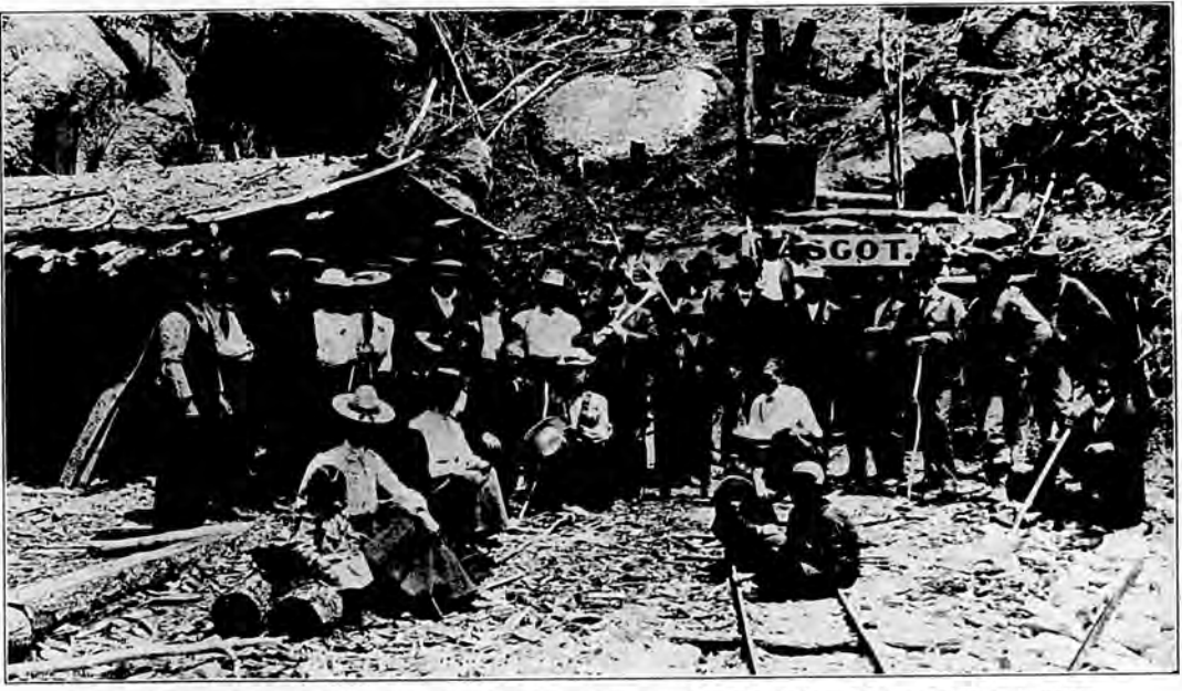
Portal of Mascot Tunnel With Senator Mason, Commander Young and Dr. Stringfield and Group of Eastern Investors.
