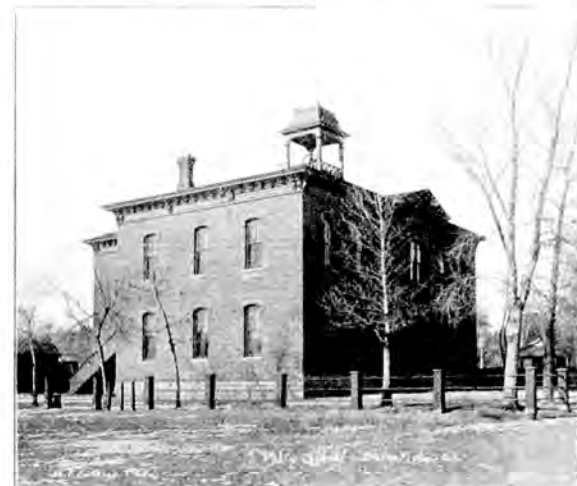
Buena Vista School Building.
