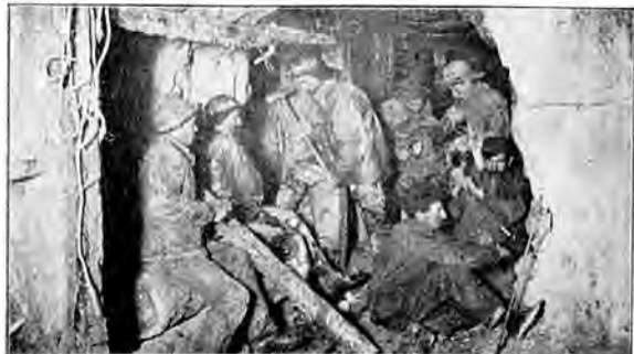
The 300-Foot Level, Jasper Mine.
