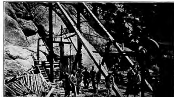
Hoisting Machinery, Jasper Mine.
