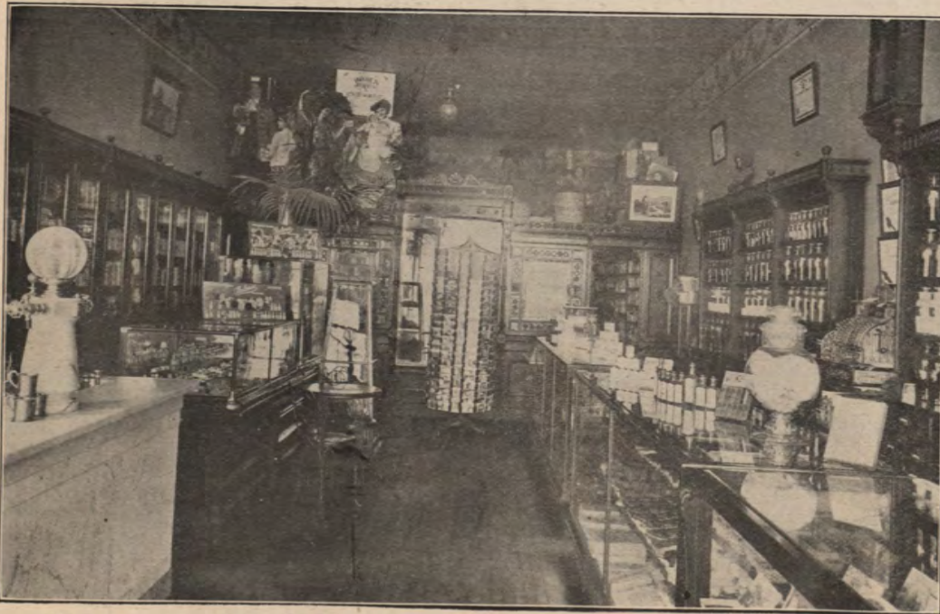
Interior view of T. C. Bode's Drug Store, corner of F and First Streets. Prescriptions are right if put up by Bode.
