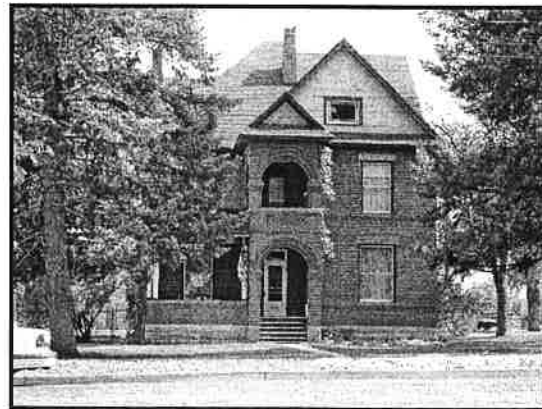
Figure 21. Area 3. 99 Poncha Blvd.
