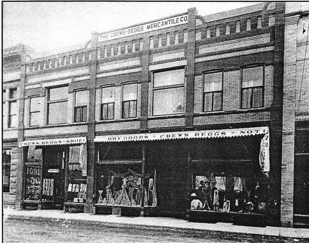
Figure 6. The first of three buildings housing by the Crews-Beggs Mercantile Company was this 1900 building at 207 F Street. SOURCE: Collman, Trails Among the Columbine , 182, Steve Frazee Collection.
