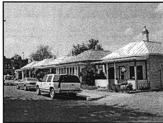
Figure 17. Area 1. 100 block of E. 4th Street.
