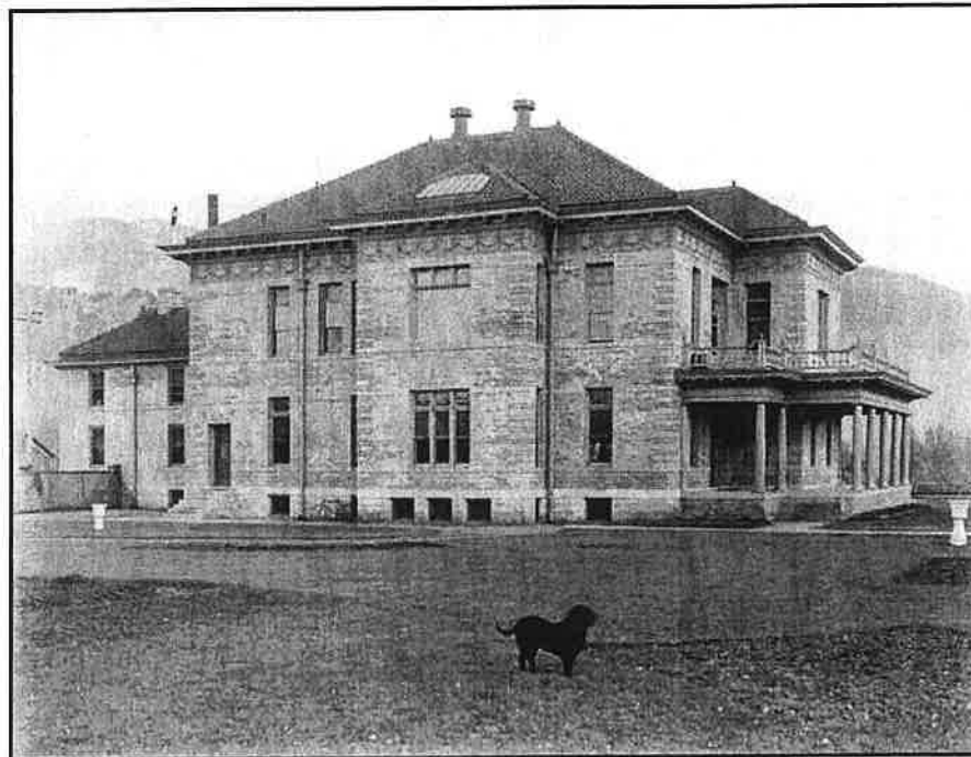
Figure 7. A new Rio Grande Railroad Hospital was constructed on East First Street in 1900, using the foundation of the building that burned. The hospital was one of the important landmarks in the northeastern part of the city, and several people who lived in the survey area worked there. SOURCE: Denver Public Library, Western History and Genealogy Department, Meigs photograph, image number X-13357, undated.
