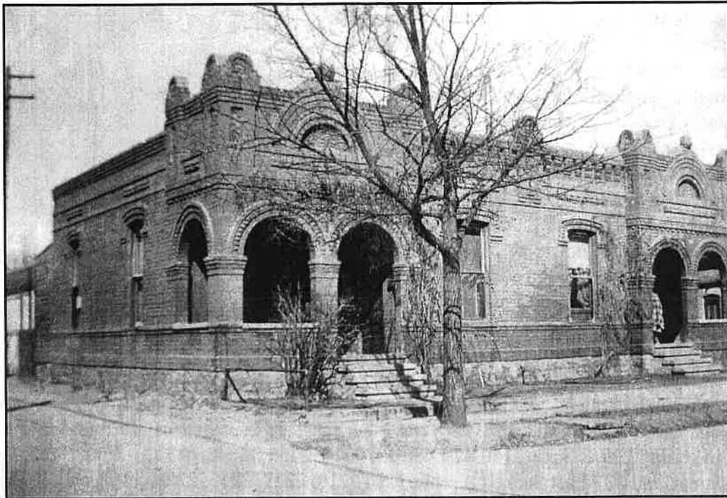
Figure 20. The Parlin Terrace, 120-22 C Street (5CF2216), was erected in 1909-10 and is an excellent example of the Terrace Type in the survey area. SOURCE: Salida Regional Library, Chaffee County Assessor, appraisal card collection, 23 February 1937 photograph.
