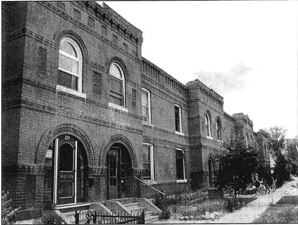
223-49 E Street, Comstock Terrace/Carpenter Terrace, 5CF2247 (1903).
