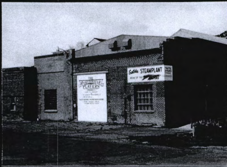
Steam Plant South Side 11-1992
