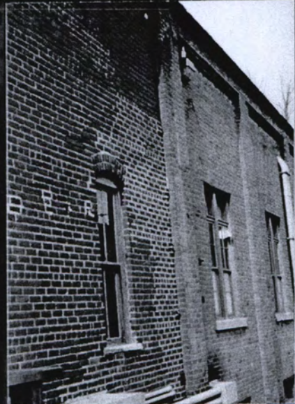
Steam Plant East wall 11-1992
