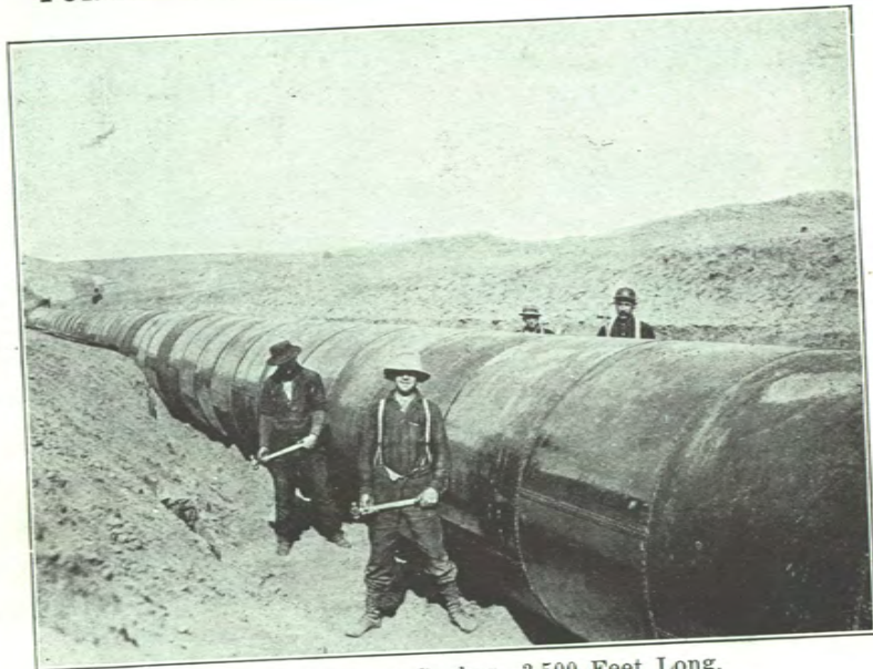
72-Inch Inverted Syphon, 3,500 Feet Long.
