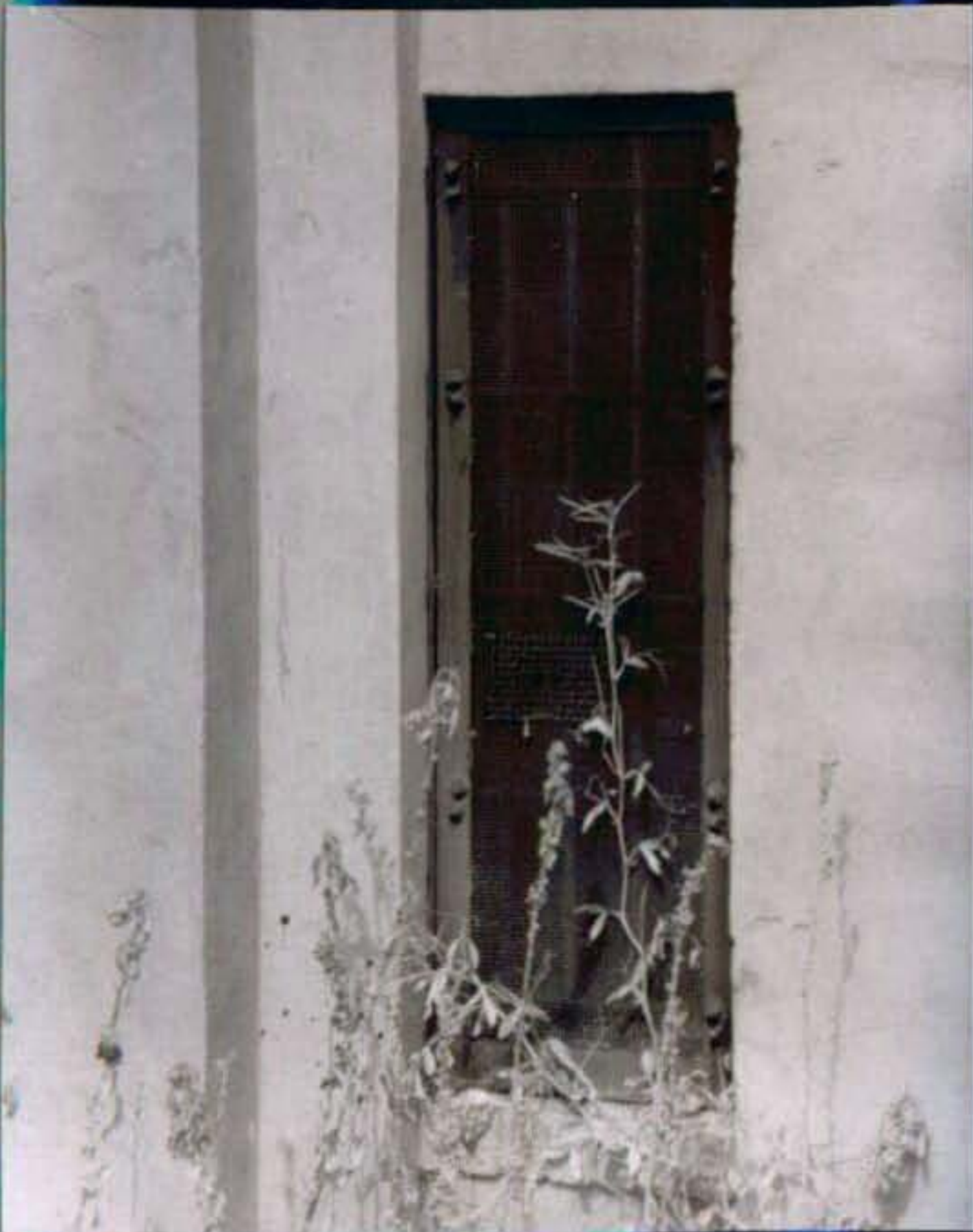
Jail Window Basement EAST CORNER 1996
