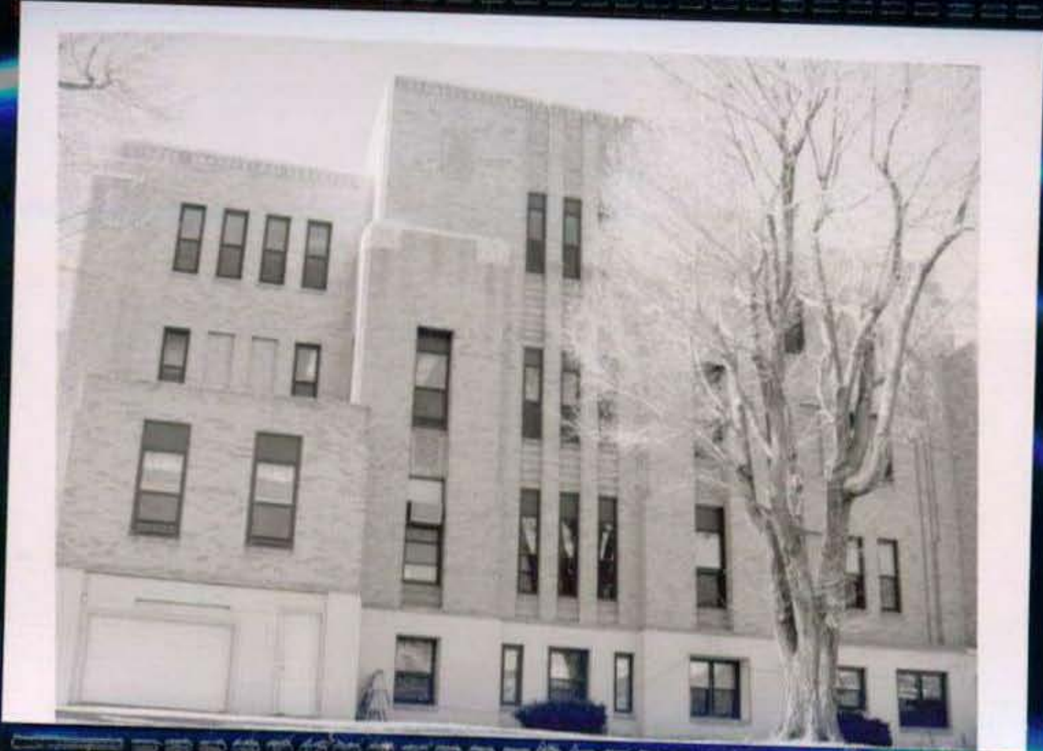
Rear elevation of Original Buildings 1996
