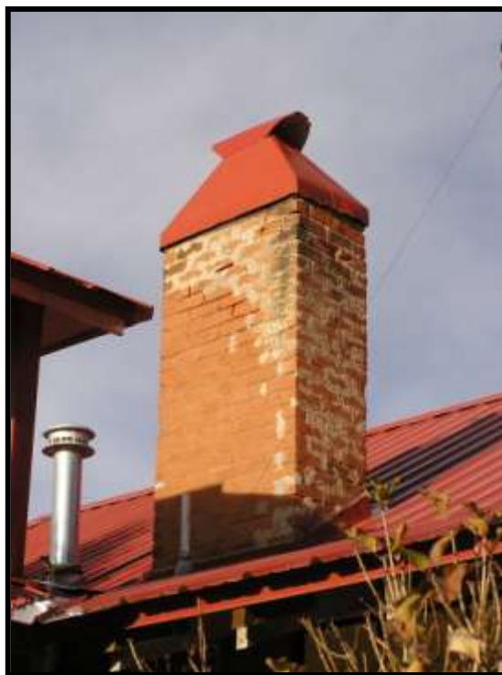
Figure 28. Chimney with red painted steel cover, looking northeast.
