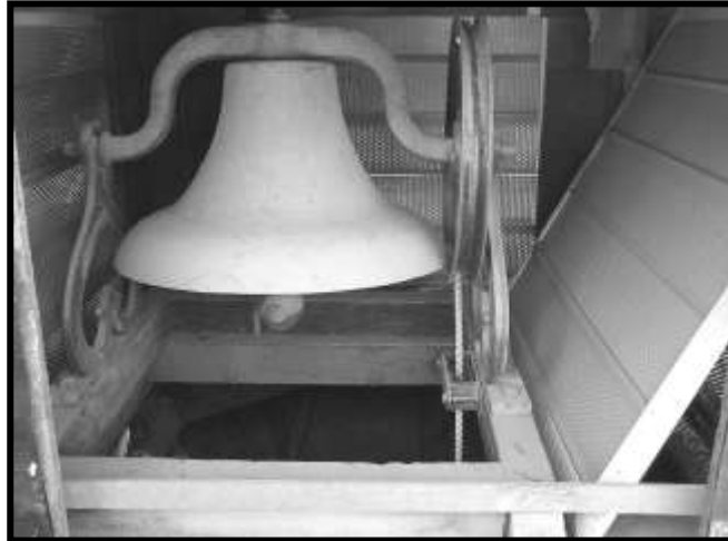
Figure 21. Bell in belfry, looking east.
