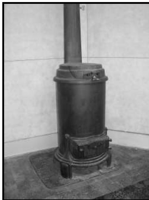
Figure 61. Wood stove in niche in South Classroom.
