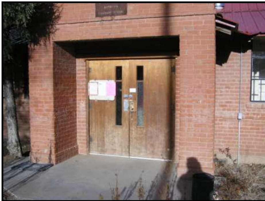
Figure 39. Entrance doors. Looking east.
