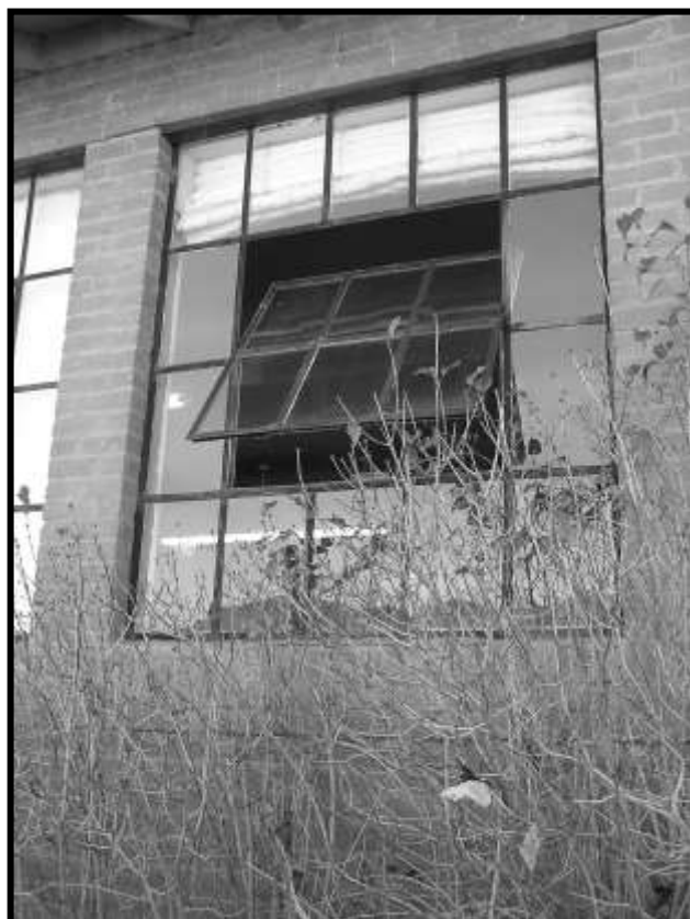
Figure 47. Window, east façade with pivoted sash in open position
