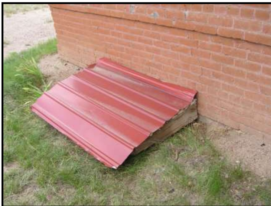
Figure 13. Crawl space entry cover. West wall, looking northeast
