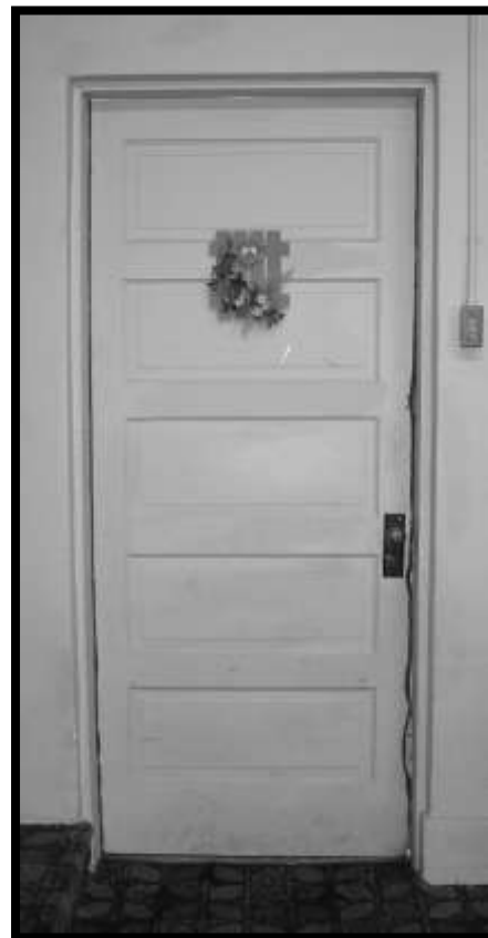
Figure 42. (right) Door leading from south classroom to hall. Typical of the three other 5-panel doors in the school. Facing west.
