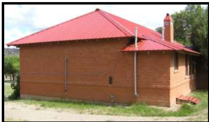
Figure 10. North façade of Coaldale School, looking south.
