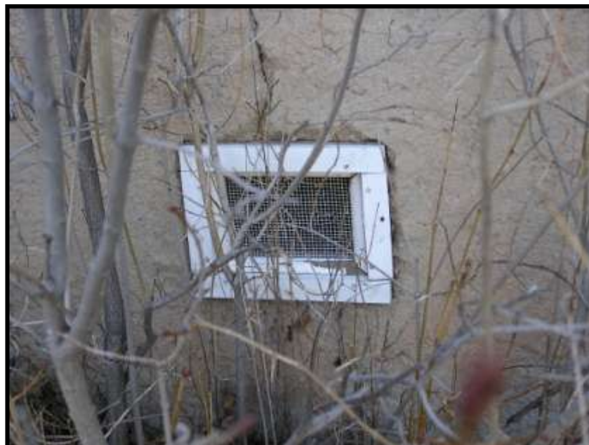
Figure 2. Crawl space vent, east foundation wall.
