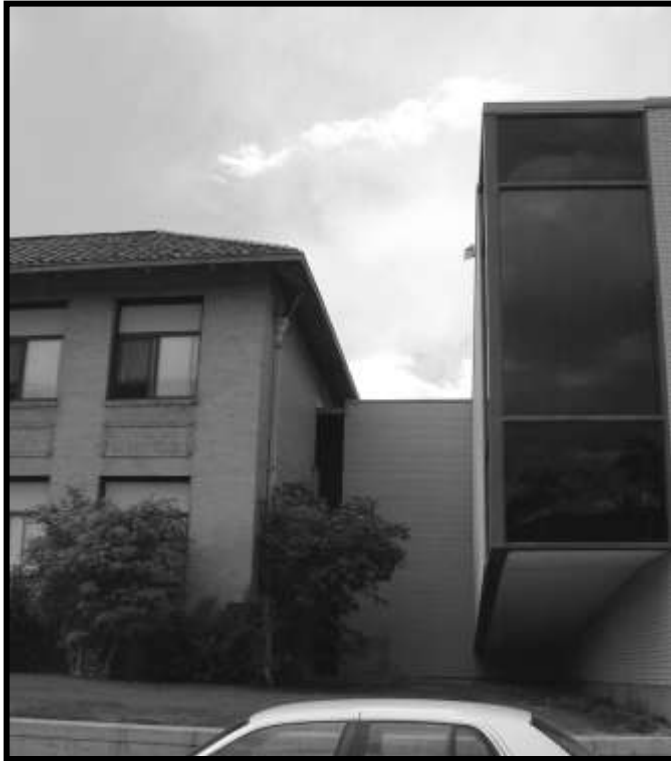
Figure 16. Northeast corner of Kesner Building. Note connector between Kesner Building and Melien Hall (to the right.)
