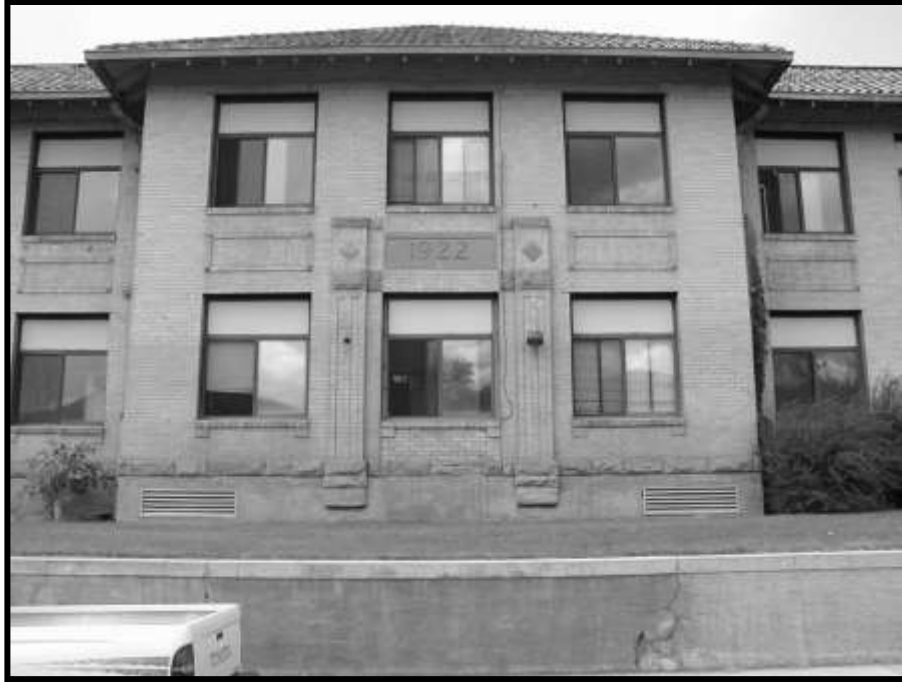
Figure 29. Decorative brick at pavilion projection (east façade).
