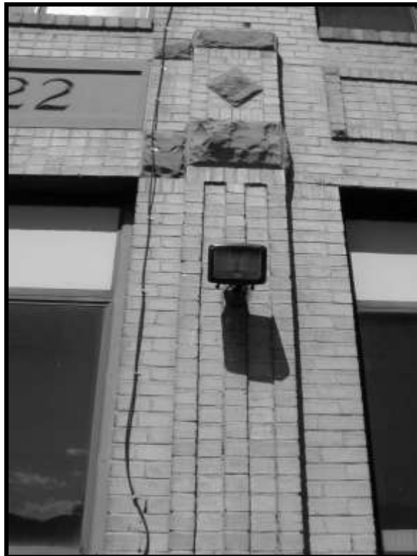
Figure 30. Brick decoration adjacent to original east building entry. Looking west.
