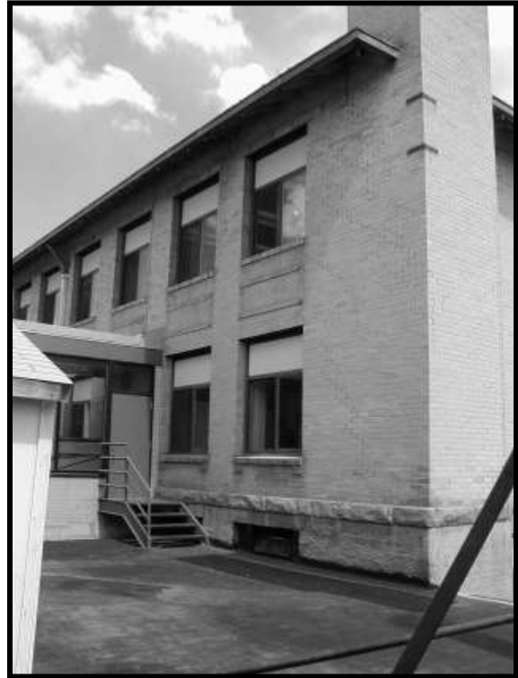
Figure 41. Stair from boiler room deck to connector. Looking northeast
