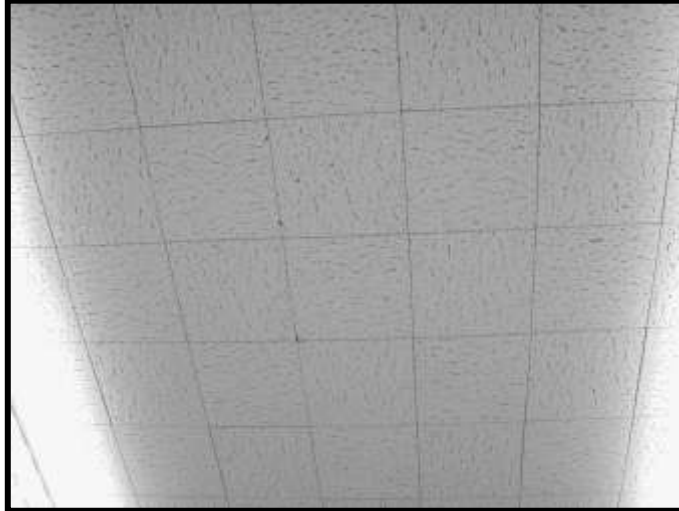
Figure 77. 12” x 12” ceiling tile with random pattern, typical of all classrooms.
