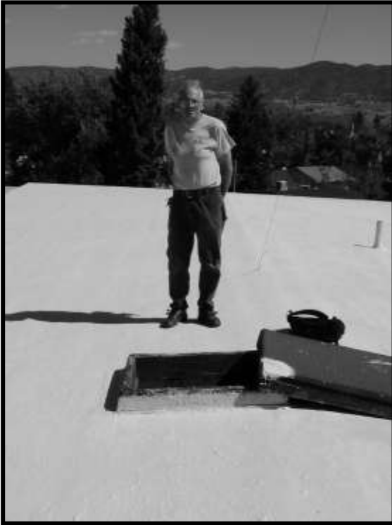
Figure 42. Frank Orzechowski on newly coated semi-flat upper roof.
