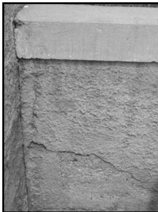
Figure 10. Retaining wall close-up.
