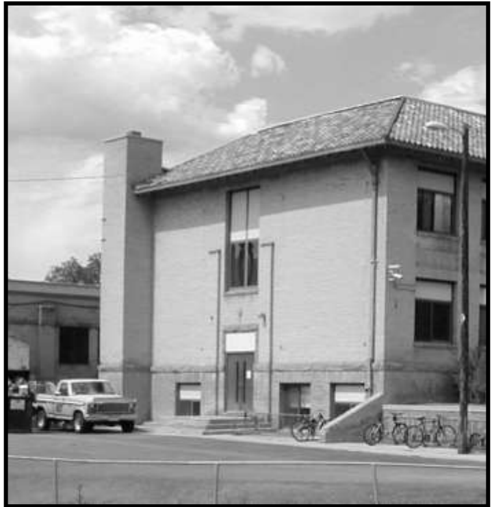
Figure 17. South façade, with Manual Training Building visible to left of chimney.
