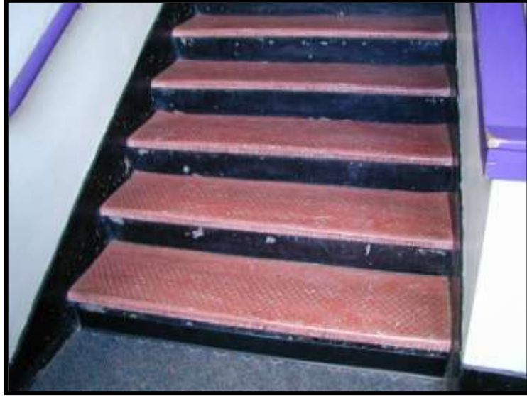
Figure 80. Second flight, south stair. Looking north.
