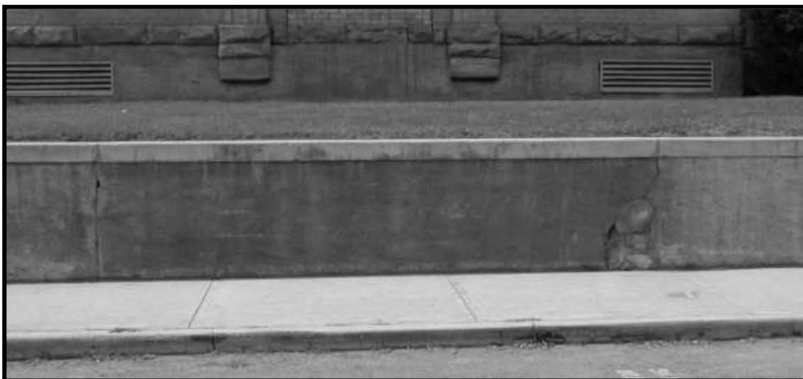
Figure 11. Concrete retaining wall infill at location of steps removed in 1962. The steps led from the parking lot up to the former main entrance level.
