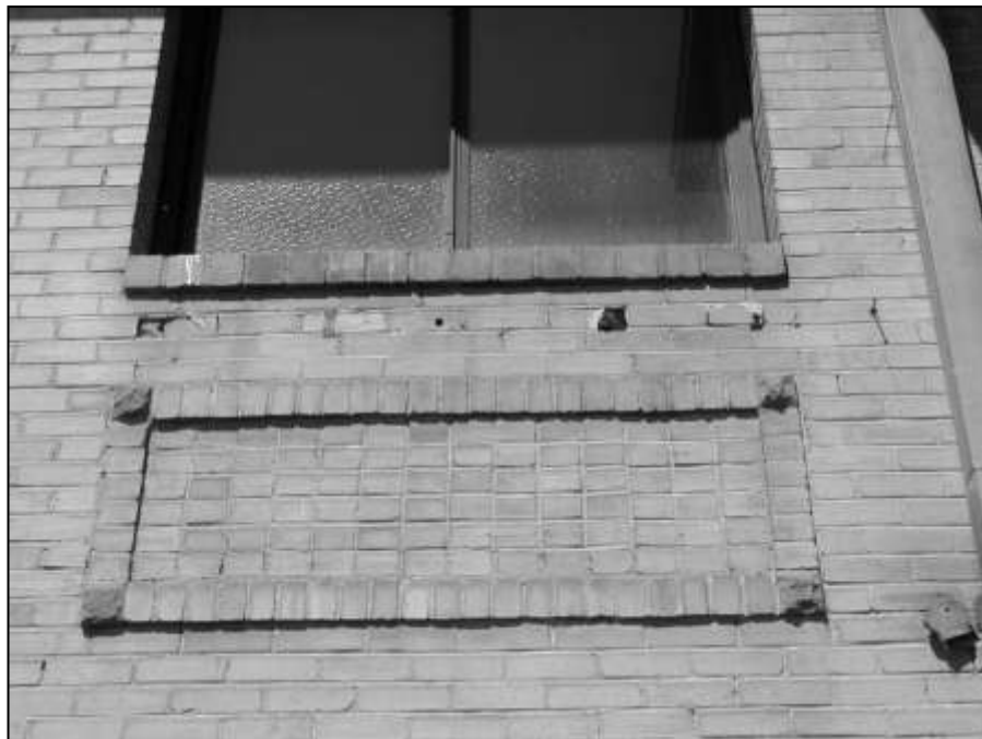
Figure 28. Decorative brick spandrel panel with sandstone bosses at corners.
