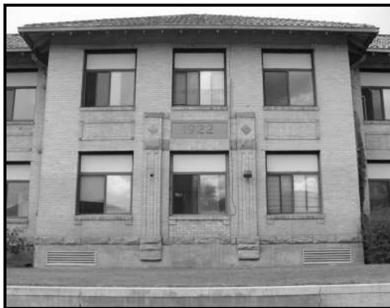
Figure 13. Central pavilion, east façade.
