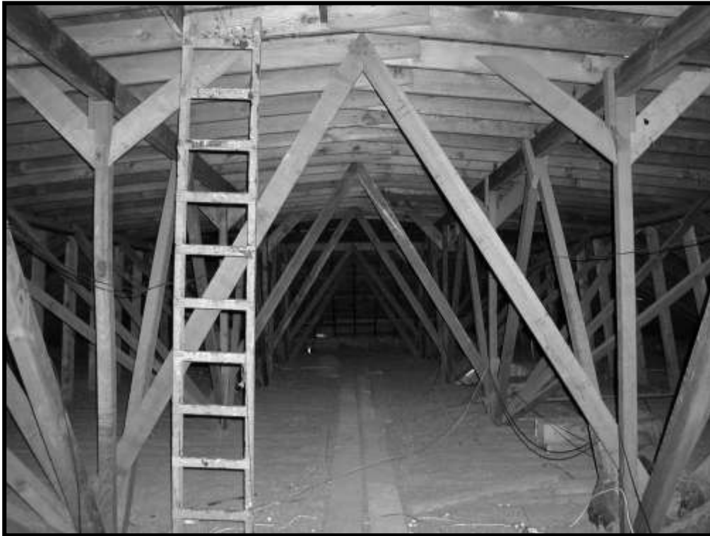
Figure 23. Attic space, looking north. Cluster of posts, struts, and braces.
