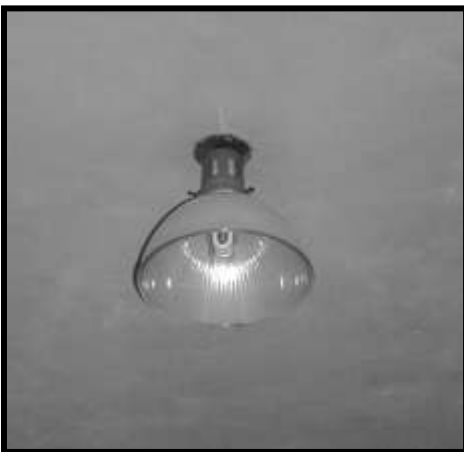
Figure 86. Original light fixture in the janitor's supply closet.
