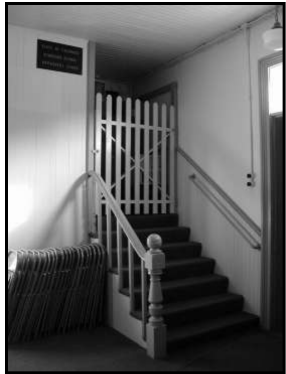
Figure 56. East Stair, looking southeast. Note black sign at top of wall to left of stair.
