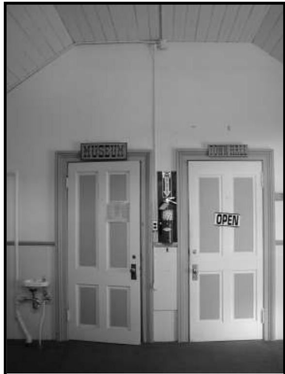
Figure 37. Doors to Town Hall (right) and Museum (left). Looking north.
