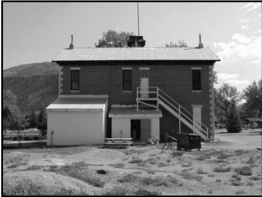
Figure 8. North façade. Note fire escape and upstairs exit door. Also note Storage Room in center below, and vault/Office to the left.
