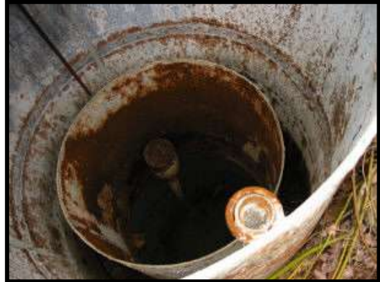
Figure 67. Interior of generator shown at left. (Photo by Robin DeLoria.)
