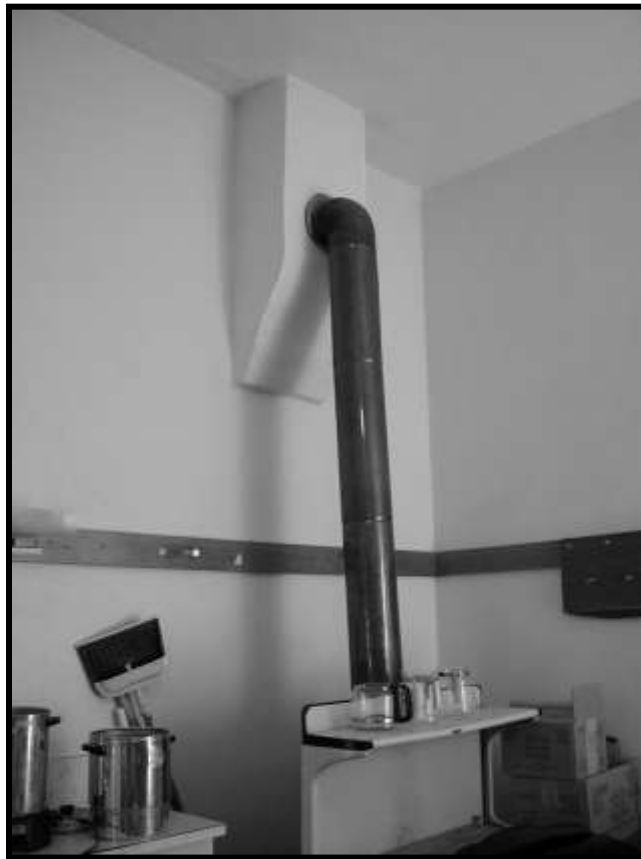
Figure 30. Stovepipe in east wall of Kitchen into retrofit chimney. Looking southeast.
