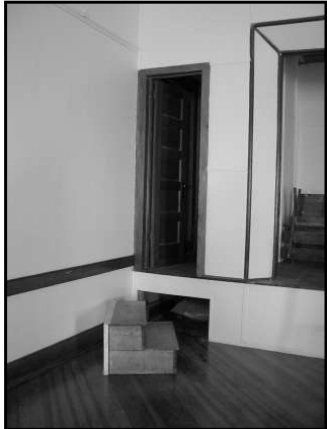
Figure 60. Steps up to south wing of the Stage.
