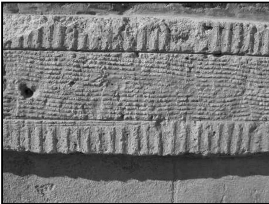
Figure 25. Close-up of watertable tooling.
