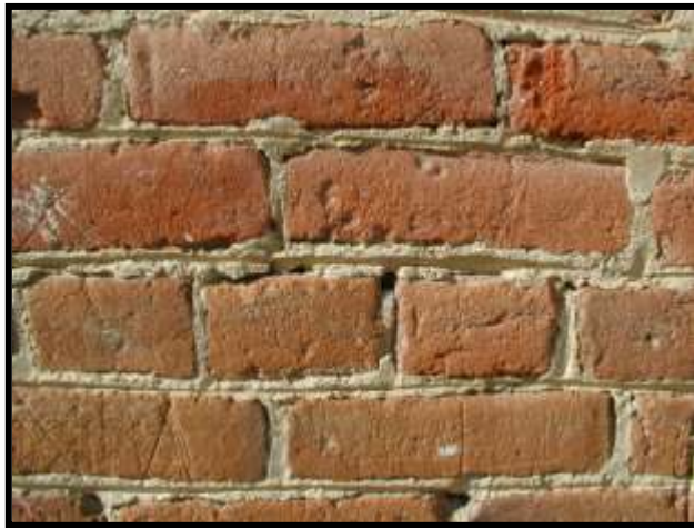
Figure 14. Grapevine brick pointing.
