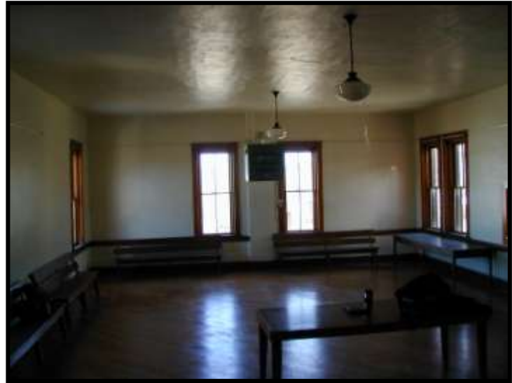
Figure 7. Auditorium, looking east from Stage. Note light fixtures, and heater suspended from east end of ceiling.
