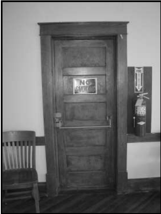
Figure 38. Five-panel door. Exit door from Auditorium, looking north.
