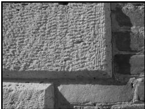
Figure 18. Quoin tooling, long face.
