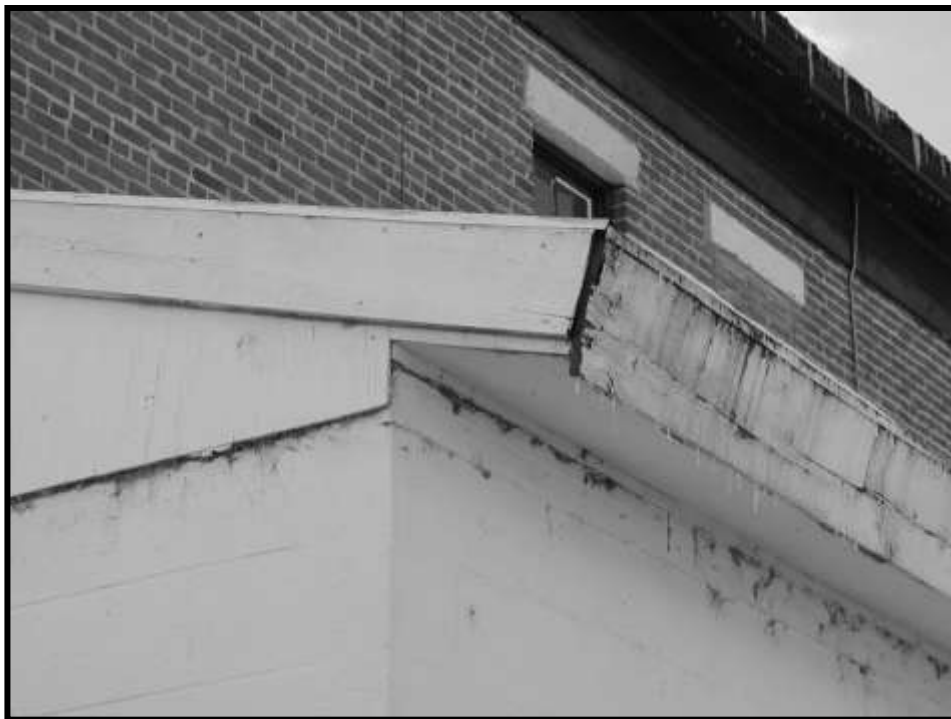
Figure 32. Vault fascia. Northeast corner, looking southwest.
