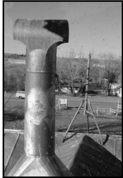
Figure 36. Tipped roof antenna, to right of chimney cap. Looking north.
