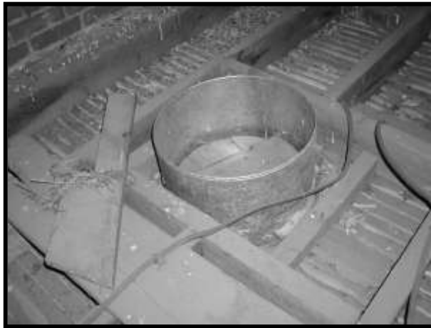
Figure 20. Pipe at ceiling penetration.
