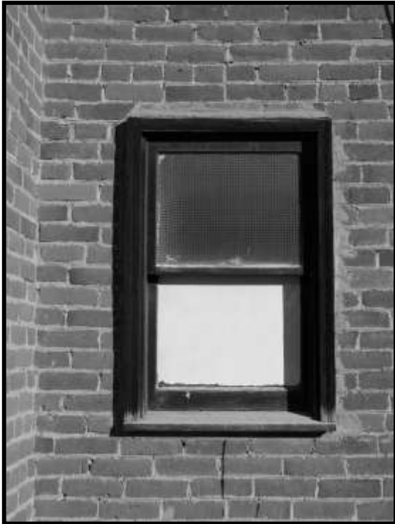
Figure 42. Girls Room window from exterior, looking east.
