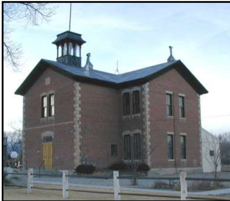
Figure 5. South and East facades. Looking northwest.
