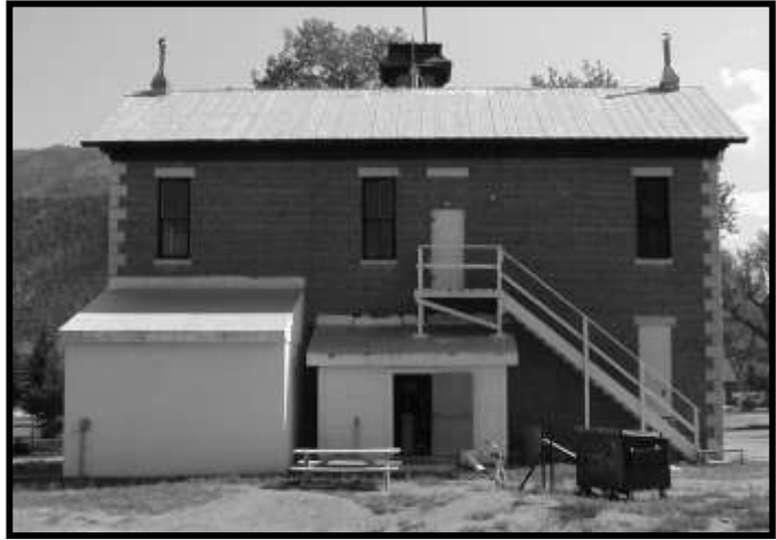
Figure 31. Rear (north) elevation, facing south. Three appendages, left to right: concrete block vault, now the Town Administrator's Office, storage shed, and exterior exit stair.
