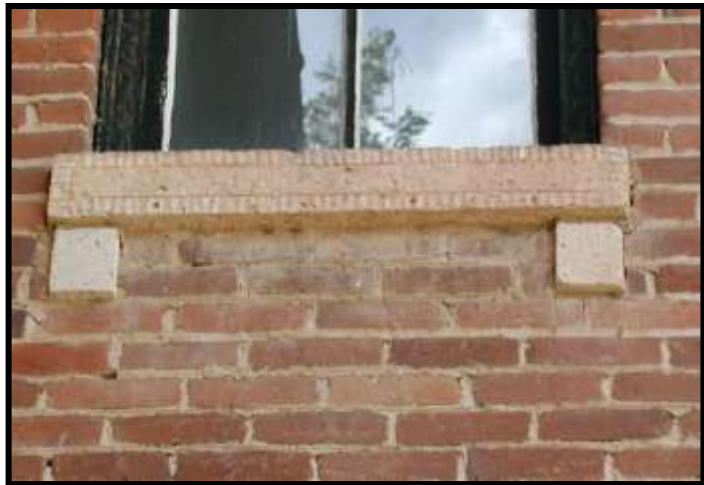
Figure 16. Window sill with dentil tool marks.
