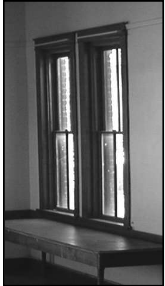
Figure 40. Interior windows, Auditorium. Looking southeast.
