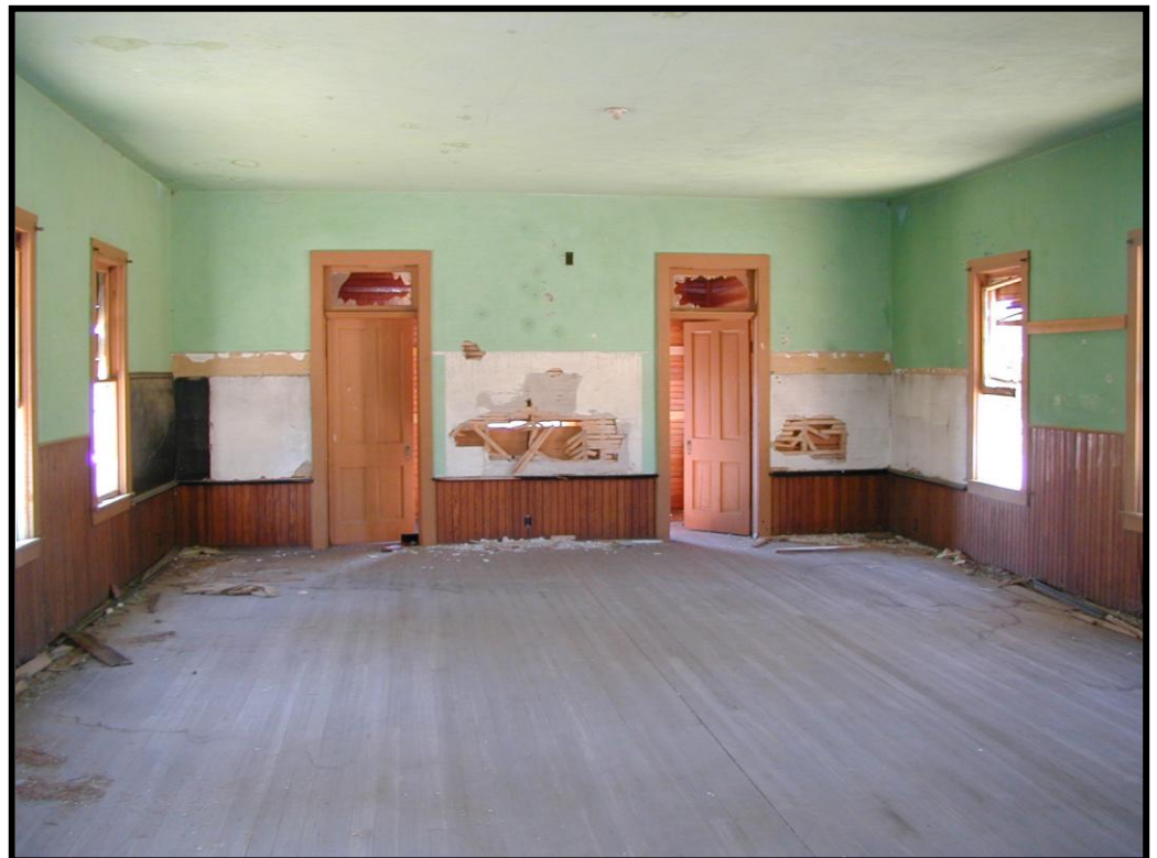
Figure 26. Schoolroom, looking south. Note four-panel doors from vestibule. Also note blackboards – extant at left, and missing at center and right.
