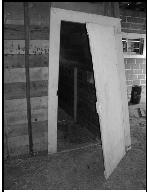
Figure 19. Door to compartments in WPA addition. Looking northwest.
