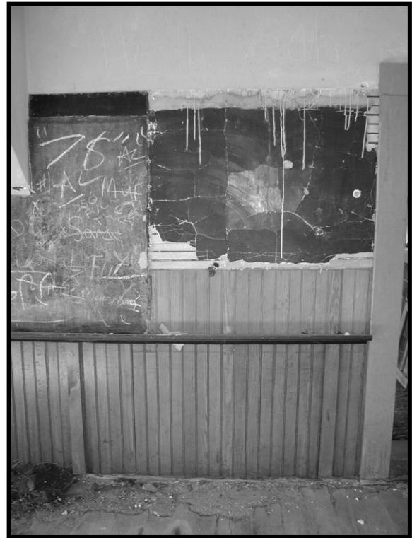
Figure 36. Blackboards. Right portion is "slating" or paint on smooth plaster. Left is either Hyloplate or a similar material.
