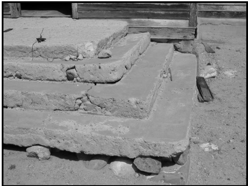
Figure 15. Front stoop. Looking north at southeast corner.
