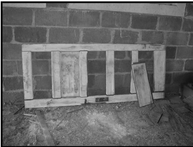
Figure 20. Probable exterior person door to WPA addition.
