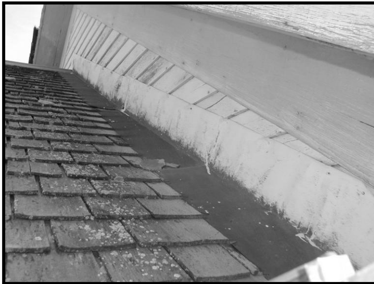
Figure 16. Vestibule roof where it joins main building. Note flashing. Looking northwest.
