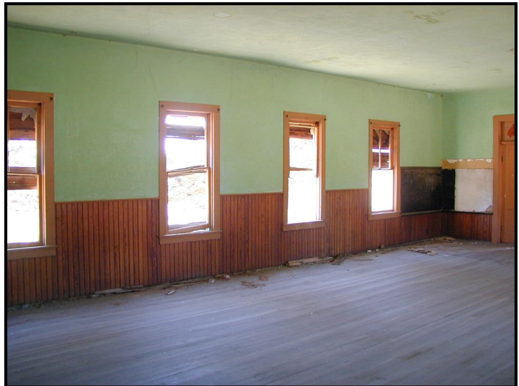
Figure 28. East wall of schoolroom, looking southeast.
