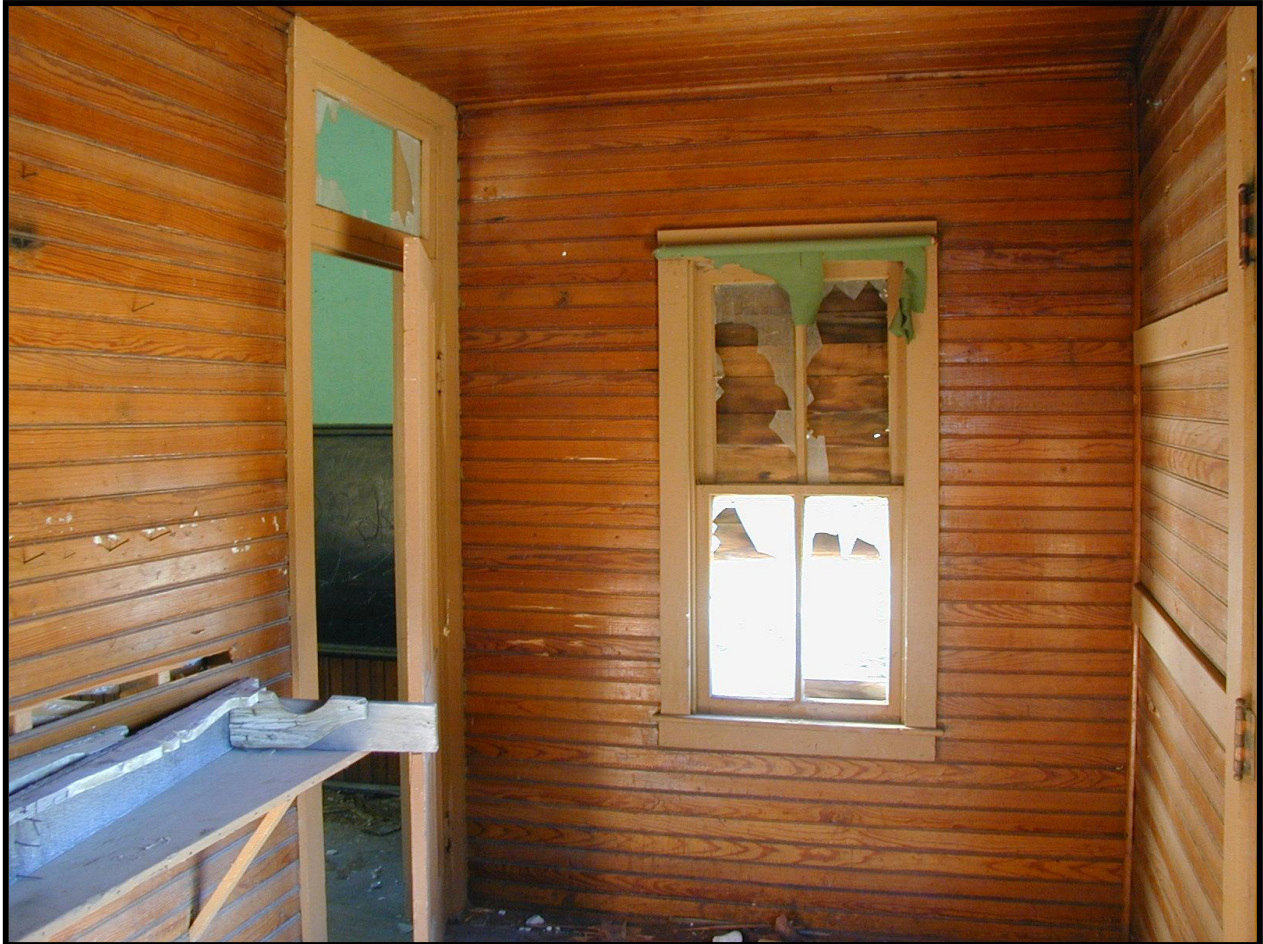
Figure 24. Vestibule interior, looking east. Note shelf on left, with nails above, and horizontal painted boards on right. Door with transom is to schoolroom. Hinges of entry door are visible just inside the right edge. Note remnants of green window shade.
