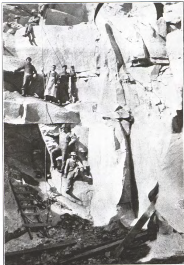
PART OF QUARRY SHOWING IMMENSE GRANITE FACE
