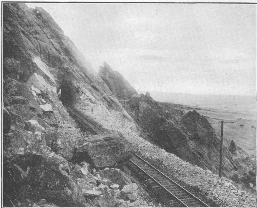
B. MOUNTAIN FRONT ON THE "MOFFAT ROAD."
