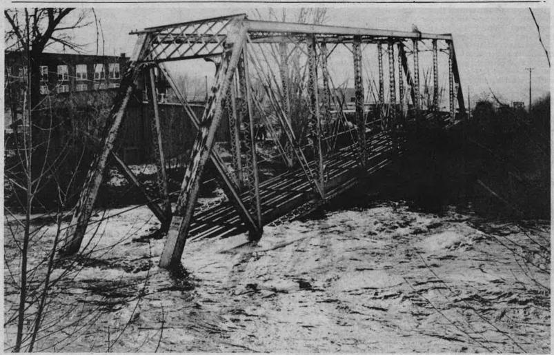
THE D&RGW BRIDGE no longer spans the Arkansas River. On Monday afternoon a railroad salvage crew, using heavy equipment, first pulled the bridge off its moorings and halfway across the river, as seen here from the north side of the river. At this point, the southern third of the bridge was cut off. That made it possible to bring the remaining twothirds out of the river with heavy equipment. Plans are to cut the bridge into 5-foot scrap pieces.
