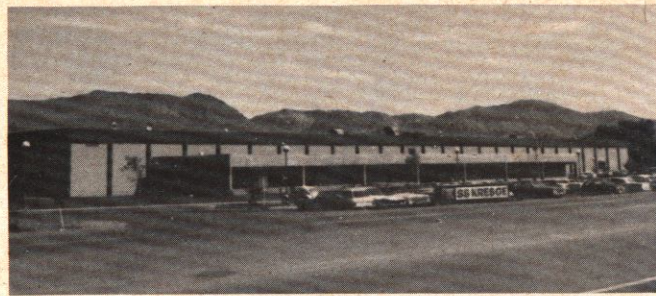
THE WESTERN DISTRIBUTING CENTER for S. S. KRESGE CO., located at Sparks, Nevada, supplies 25% of all commodities handled by the K-Mart Stores located in the eleven western states. Headquarters for S. S. Kresge Co. is located at Detroit and other distribution centers are located at Fort Wayne, Ind., and Lawrence, Kansas. The Sparks facility consists of 800,000 sq. ft. of warehouse space and plans are currently under way for a 200,000 ft. addition.
