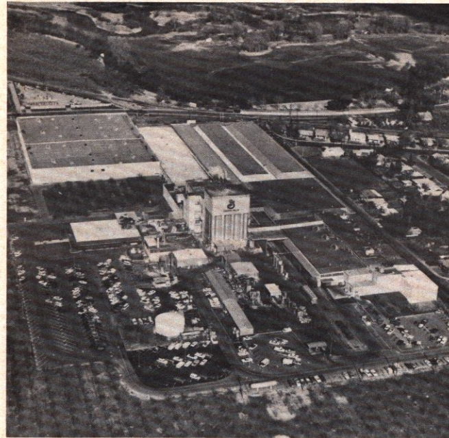
GENERAL MILLS, INC. at Lodi, California, began its operation in 1948. It is one of five General Mills Package Foods plants located in the United States. Since that date the plant has grown considerably, both in variety of products produced and in size. A mix plant has been added to keep up with the increased demand for more Betty Crocker mixes, and additional warehouse space has been added. Today the plant employs over 500 employees. Product distribution is made to all western states, Alaska, and Hawaii. This amounts to more than 5,000 railroad boxcars plus 1,800 truck loads of product shipped to these points.
