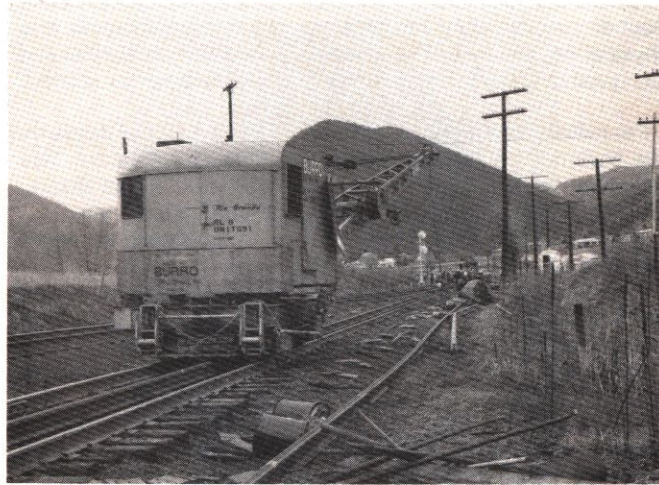
Burro crane threads new welded rail to center of track.
