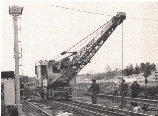
Burro crane sets out old rail.
