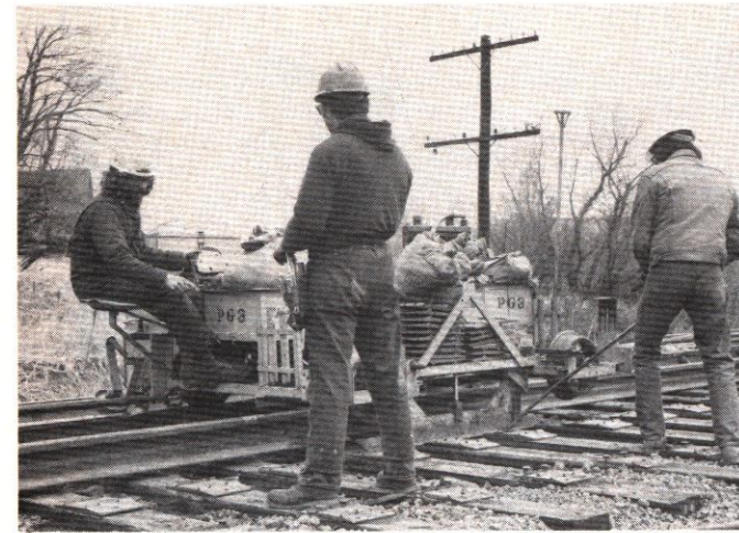
Dunrite gager and crew move in to accurate gage track width, 4'-8½"
