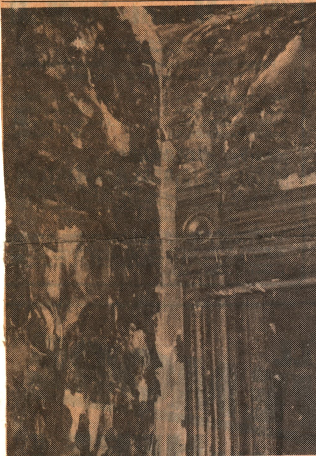
SEARING HEAT charred wood; paint; wallpaper and plaster in a flash explosion in the Ideal Rooms. This room was the only room still on fire when firemen arrived. The explosion had blown out the rest of the blaze.
