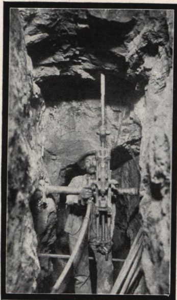
OPERATING AIR DRILL 900 FEET UNDER GROUND.
