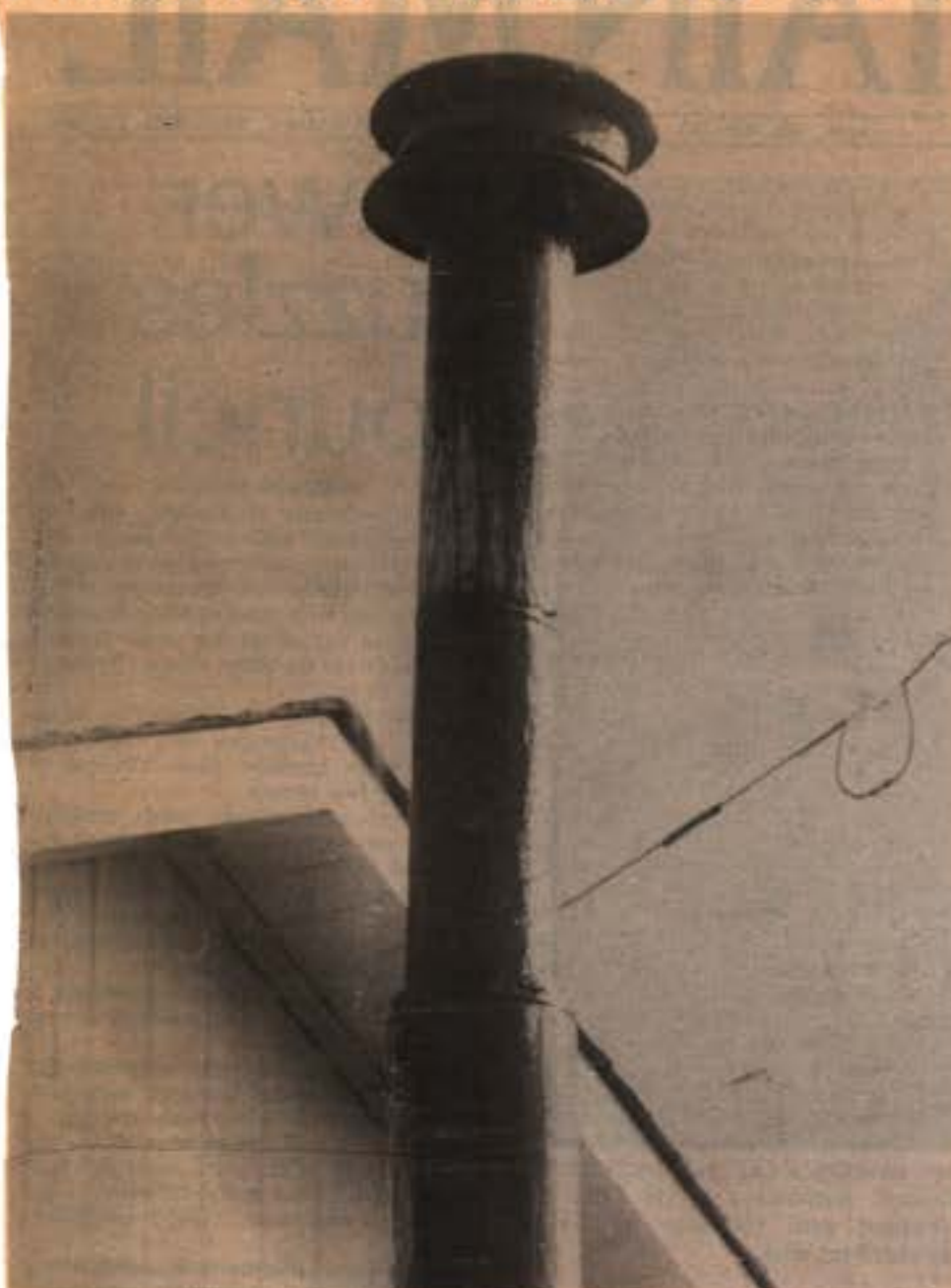
IF OUTSIDE APPEARANCES are any indication, this metal chimney is long overdue for a cleaning. You can see creosote running along the outer surface, an indication that the inside is dirty.
